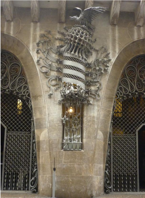
Fig. 1. Set situated in the middle of the main facade of Palau Güell. Photograph of the author.
