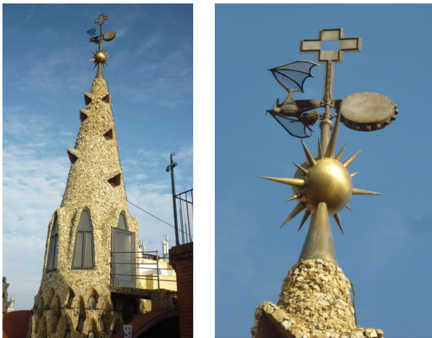
Fig. 6. Exterior of the roof spire. Photographs of the author.
